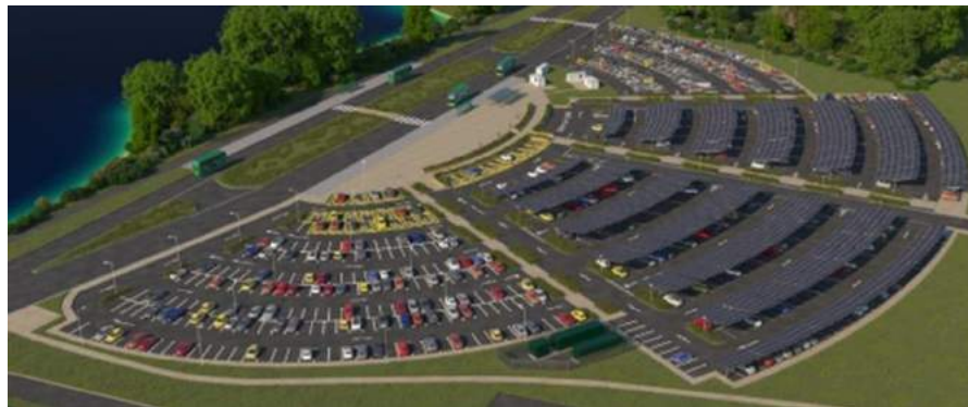
Fig 3.6 The 1MW solar farm at St Ives Park & Ride
