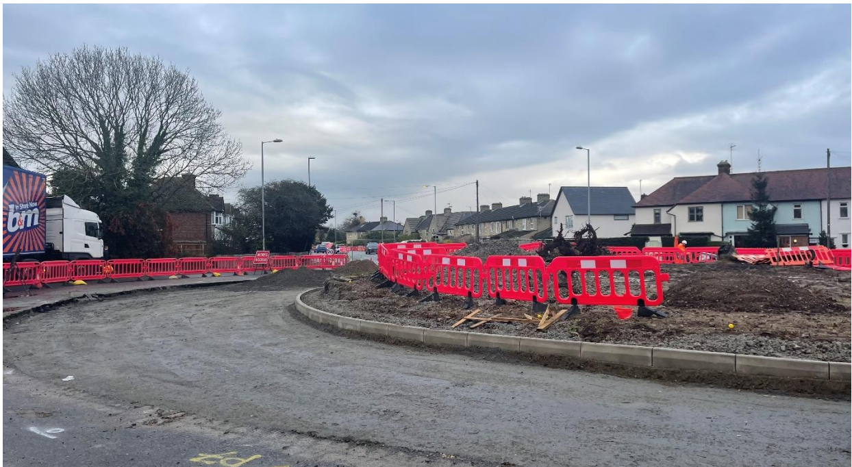
New kerb line and drainage on the Elizabeth Way roundabout
