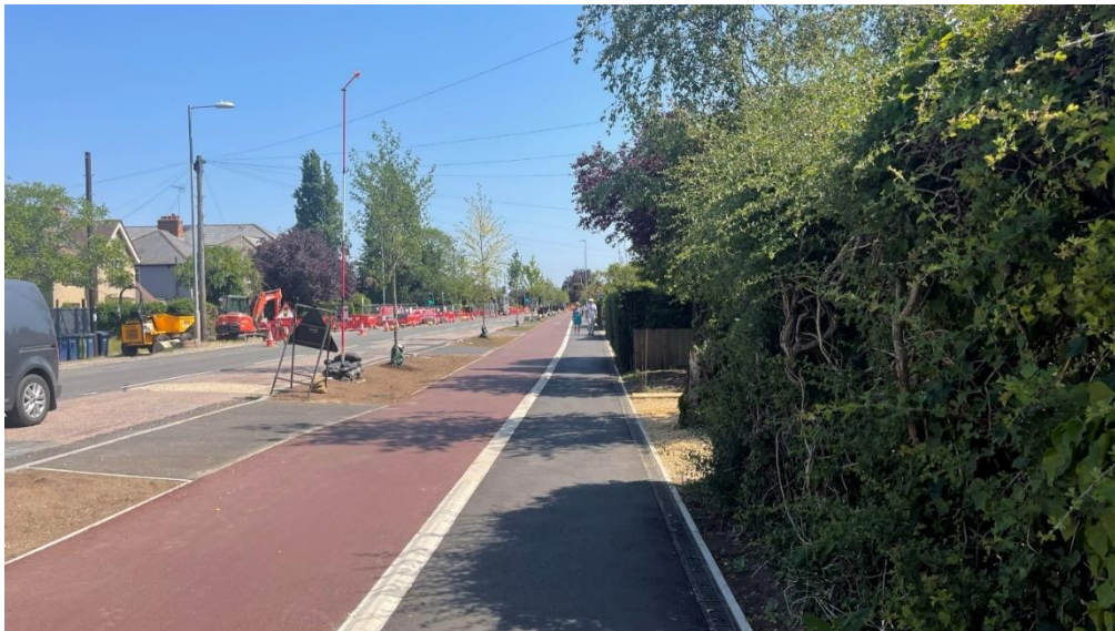
*Completed section between Fraser Road and south of Cook Close
