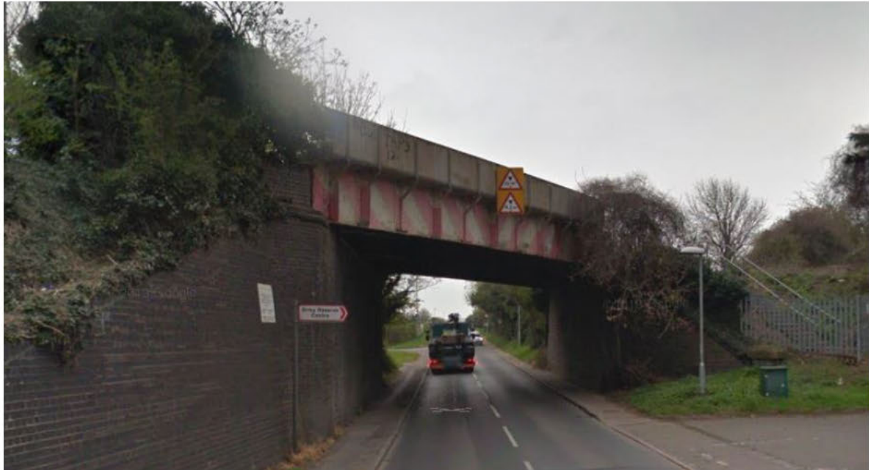
Figure 2: Railway bridge over Coldhams Lane
